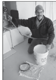
Larry Brown drains hard water sediment from a water heater
